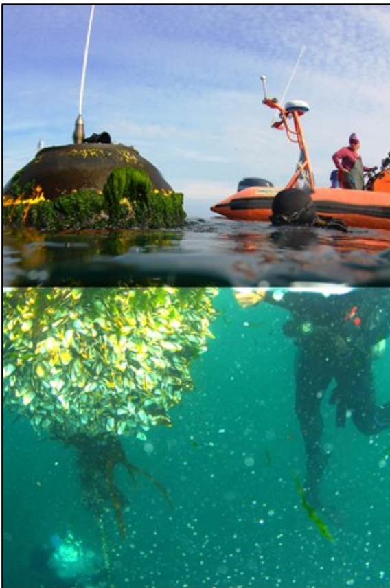
Figure 1 (c) Off the coast of California. The underwater part is encrusted by hard fouling. Courtesy of Scripps Institute (2010).
